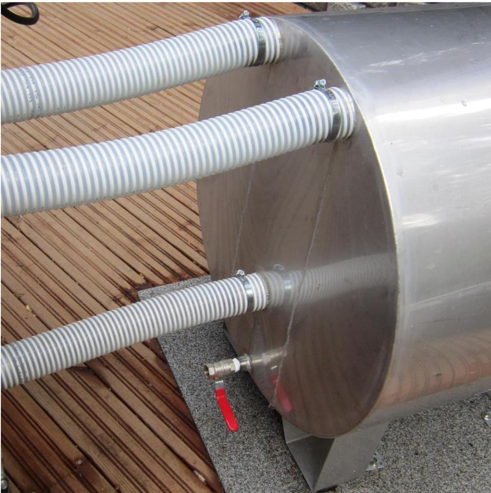
Make sure to open the water jacket tap of the stove after use. The tap is closed in this picture.
